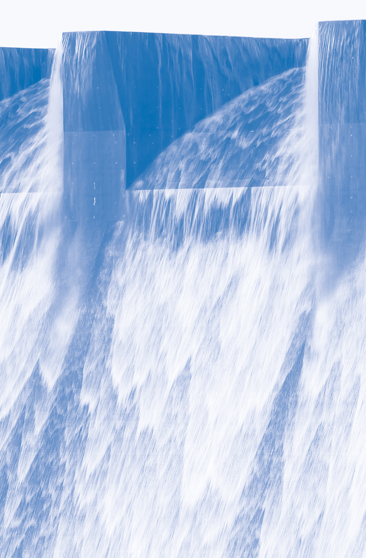
Midmar dam wall overflowing in 2009, Howick, KwaZulu-Natal, South Africa.
