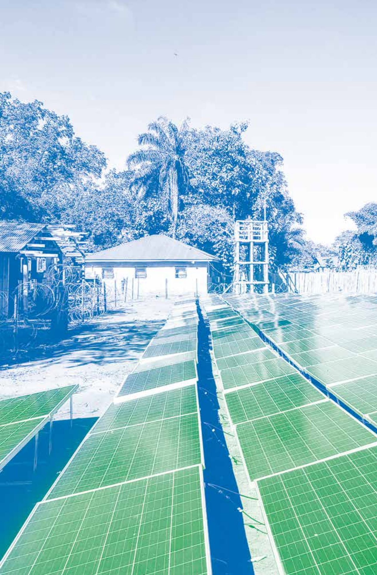
Ground mounted solar power plants in Zimbabwe.
