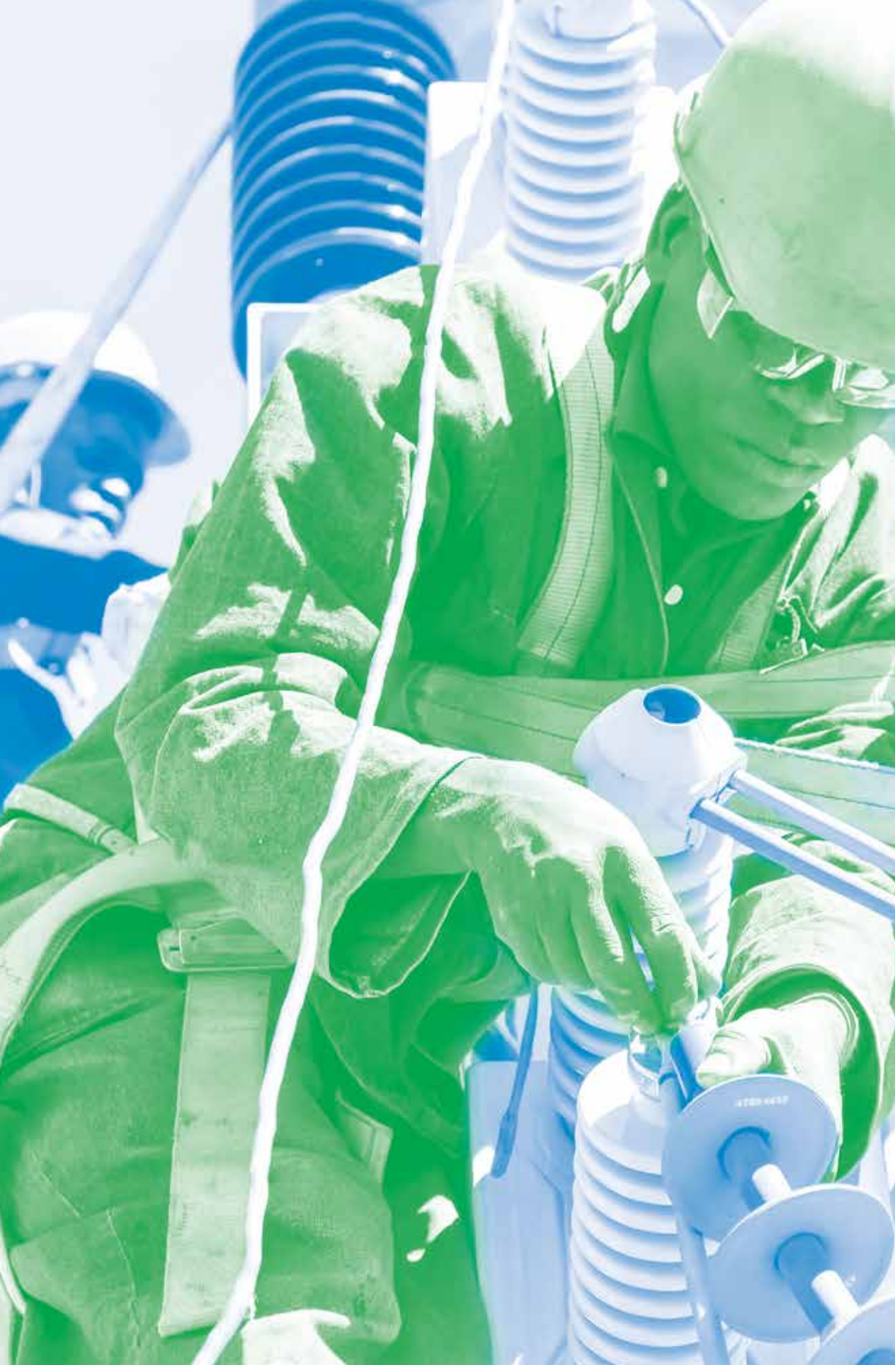
Electricians working on high-voltage power lines. Johannesburg, South Africa.
