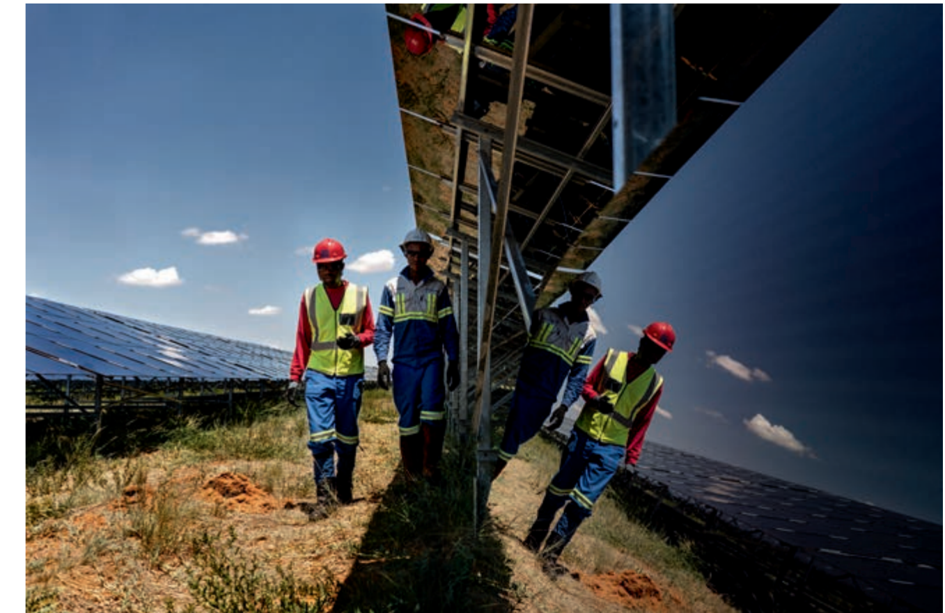
▲ Workers substituting a solar panel in Adams solar plant in Kathu, Northern Cape. ◀ Brian Galvin descending from a wind turbine that he had just repaired in Gibson Bay, Eastern Cape.
