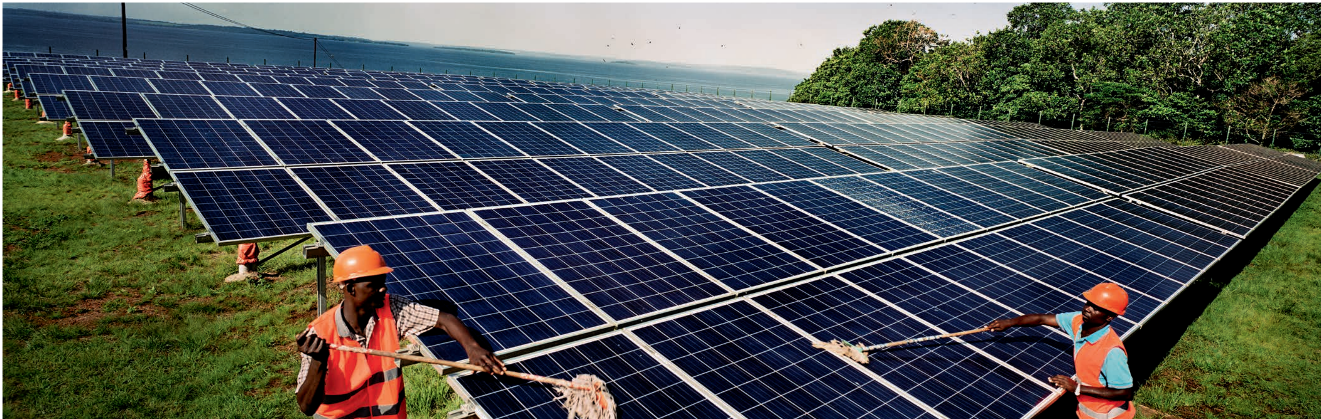
Geoffrey Mangali and Jonathan Makanga, technicians of the mini-grid ▲ of Absolute Energy, performing the routine cleaning of panels.
