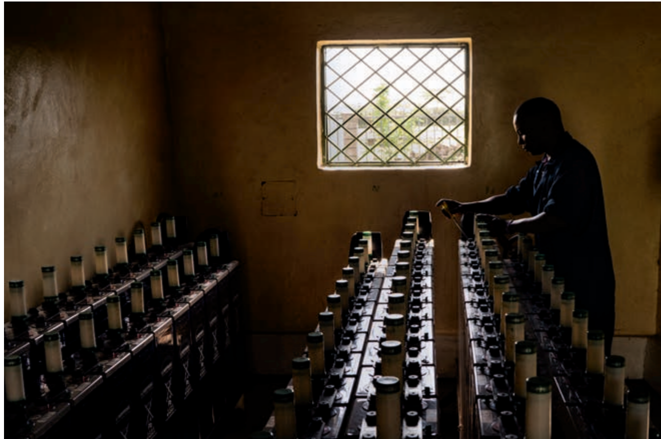
A routine control of the solar power plant's batteries in Talek. ▲
