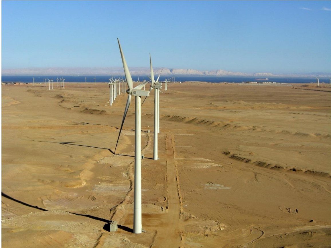
Zafarana Wind Farm, Red Sea, Egypt (360 MW), the largest wind farm on the African continent.
